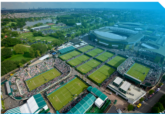
Ampetronic phased array hearing loops installed at Wimbledon, London, UK
