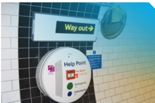
Help points incorporating Ampetronic HLS Series drivers London Underground, London, UK
