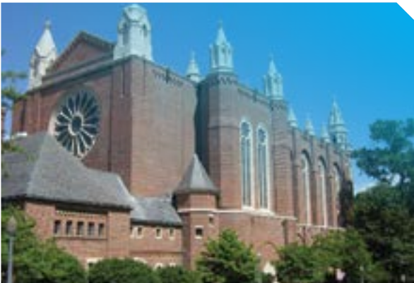
First Presbyterian Church, Greensboro, NC, USA is fitted with Ampetronic loop systems
