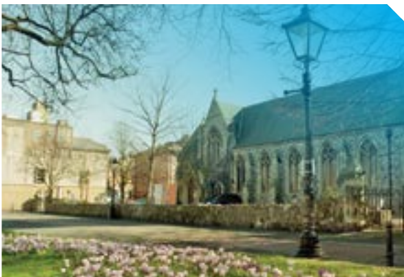
Holy Trinity Church, Southend-on-Sea, UK is fitted with an Ampetronic loop system
