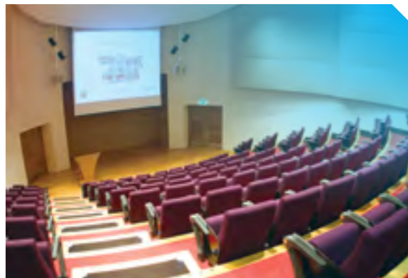
Magdalene College, Cambridge, UK utilises an Ampetronic perimeter loop
